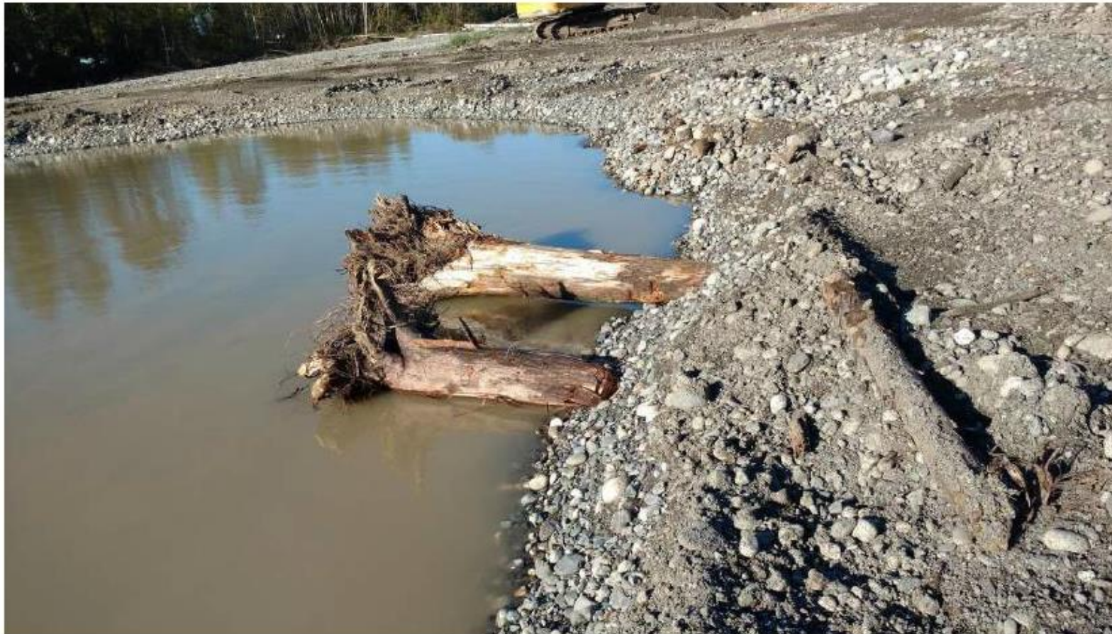
L1: LWD #L2016-1 –LWD structure placed along the bank side of the pit.
