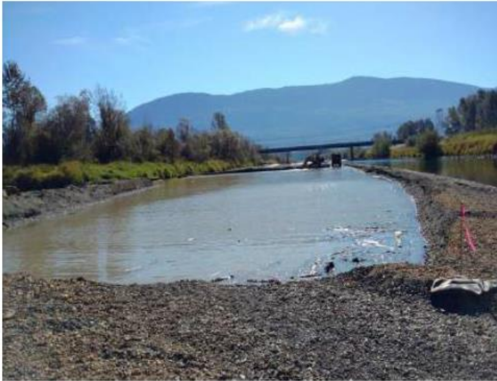
KW7: Work in progress. View from downstream end of site. September 14, 2016.
