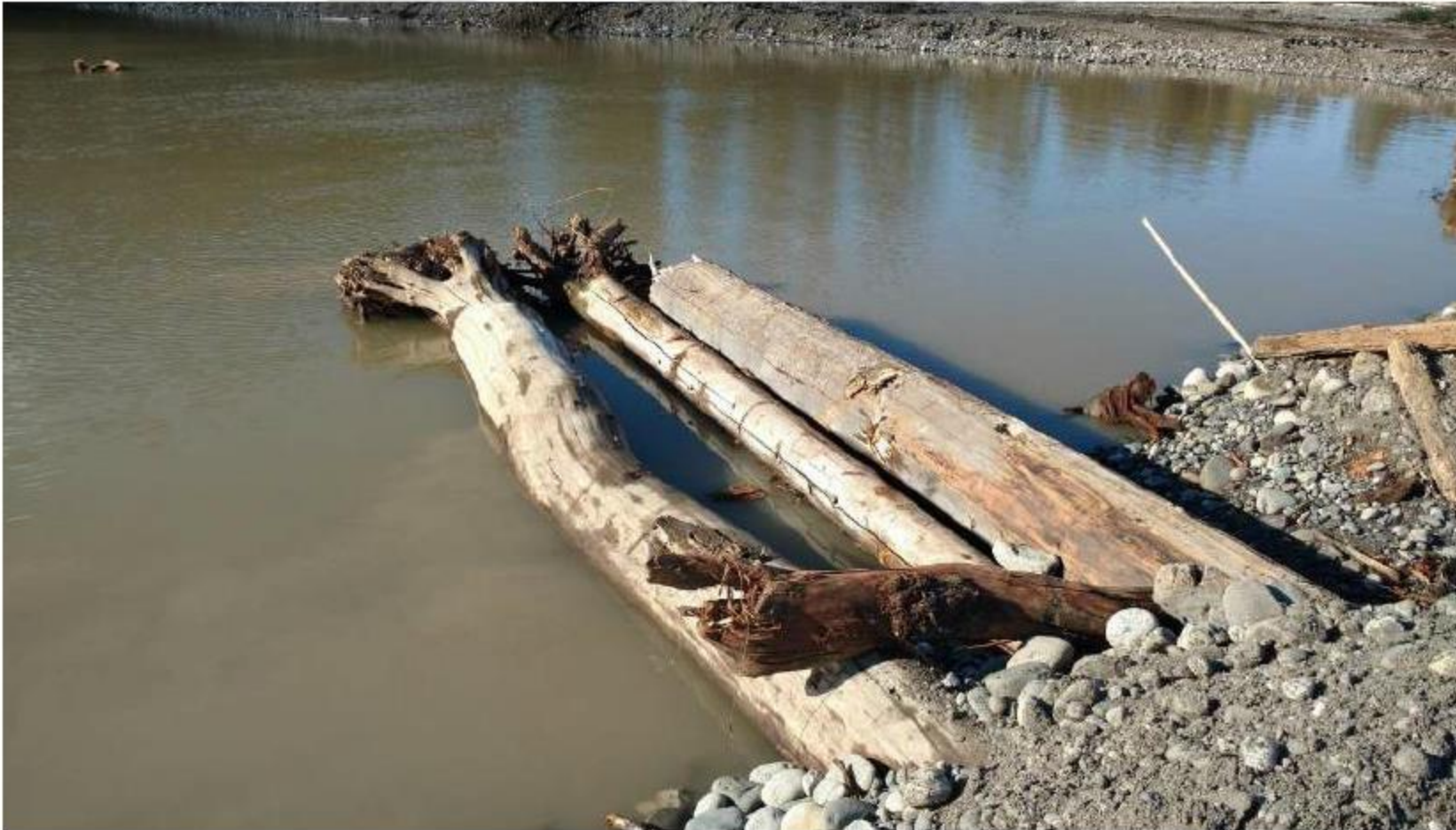
L2: LWD #L2016-2 –LWD structure placed along the bank side of the pit upstream of LWD #L2016-1.
