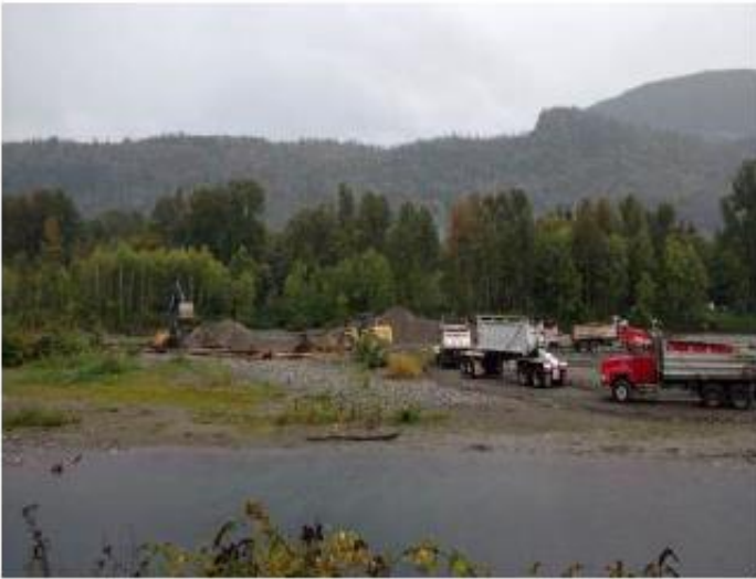
L7: Machinery on site. September 19, 2016.
