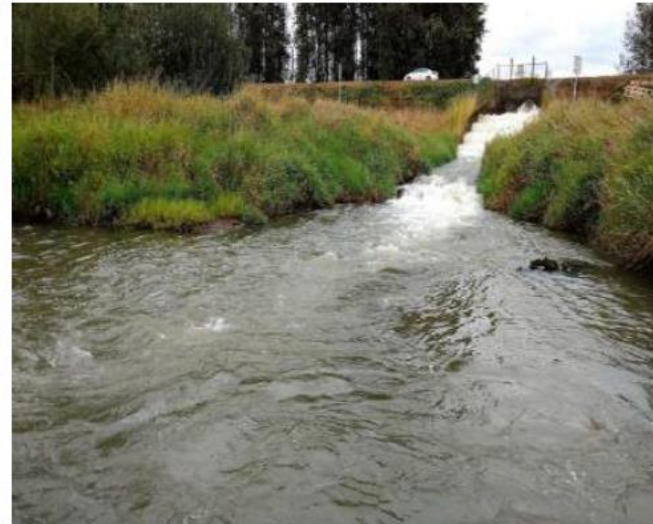
KW6: Pump station water release. September 7, 2016.
