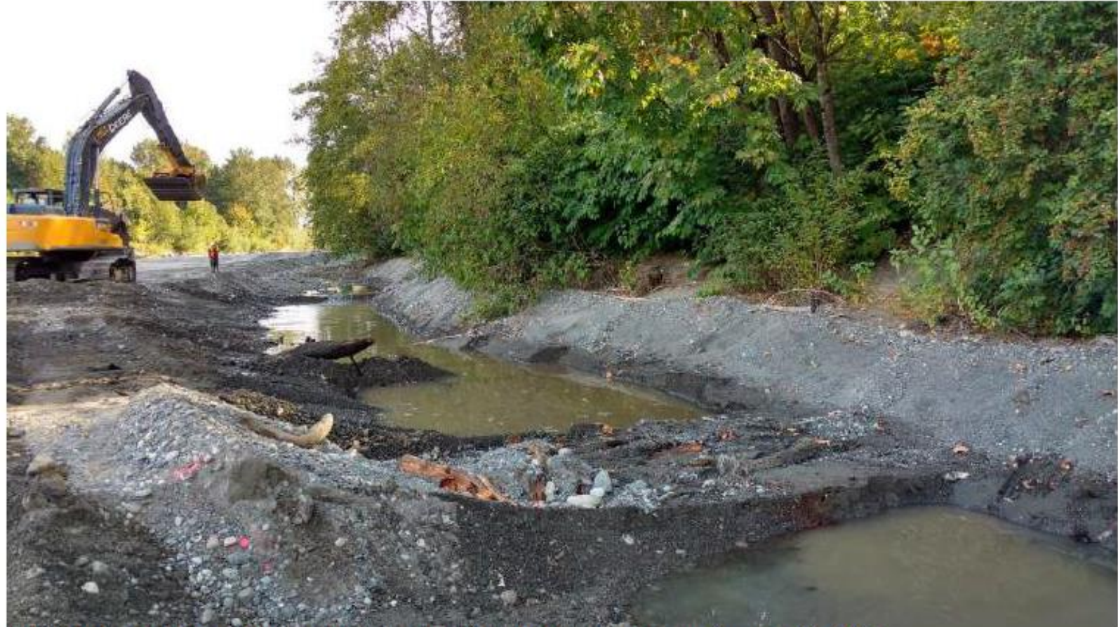
Habitat channel construction work in progress looking upstream. August 26, 2016.
