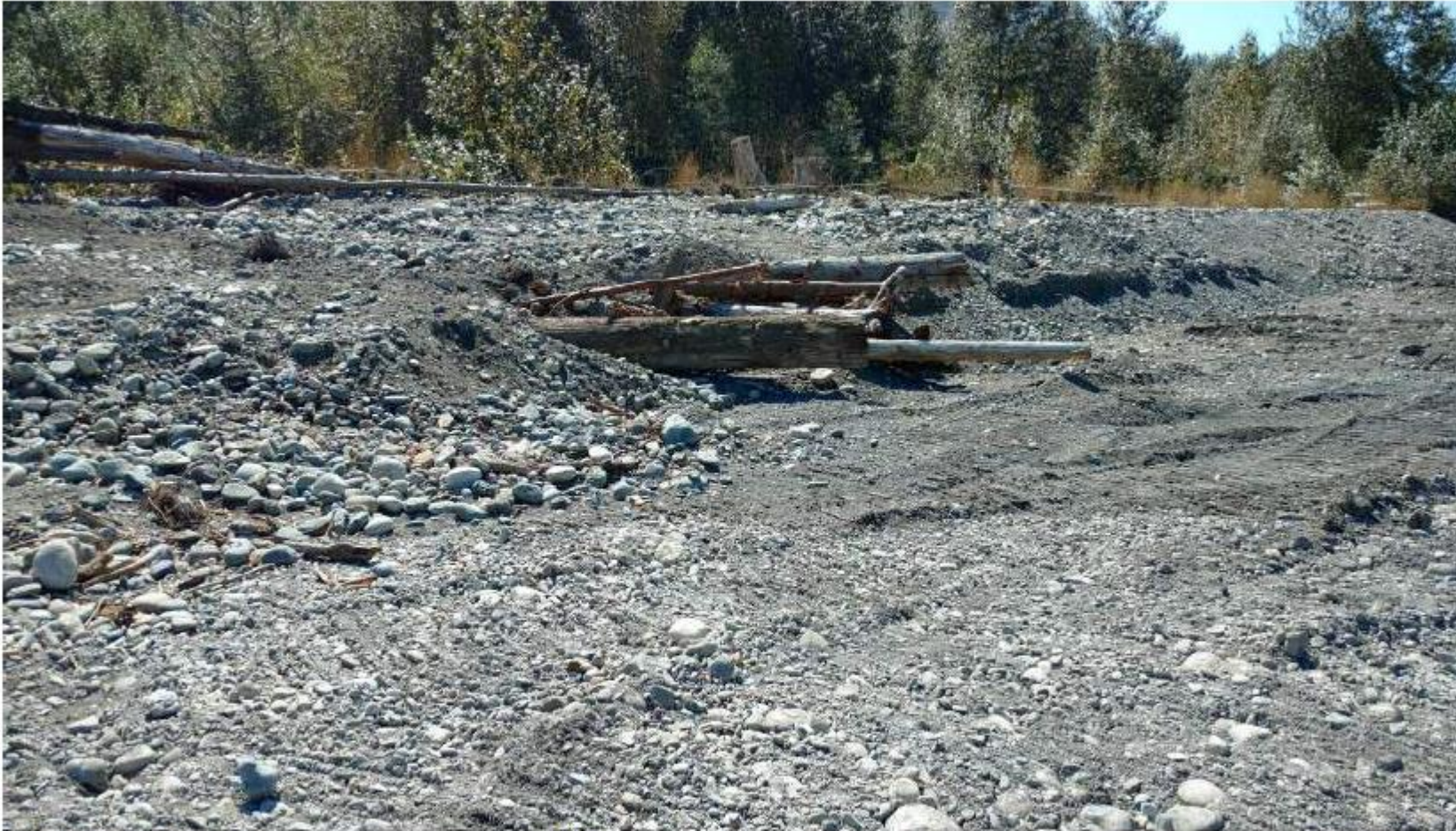
G2: LWD #G2016-2 – several pieces of LWD placed in scalded pit along the bank side. Note a platform of boulders created upstream of LWD complex to enhance fish habitat.
